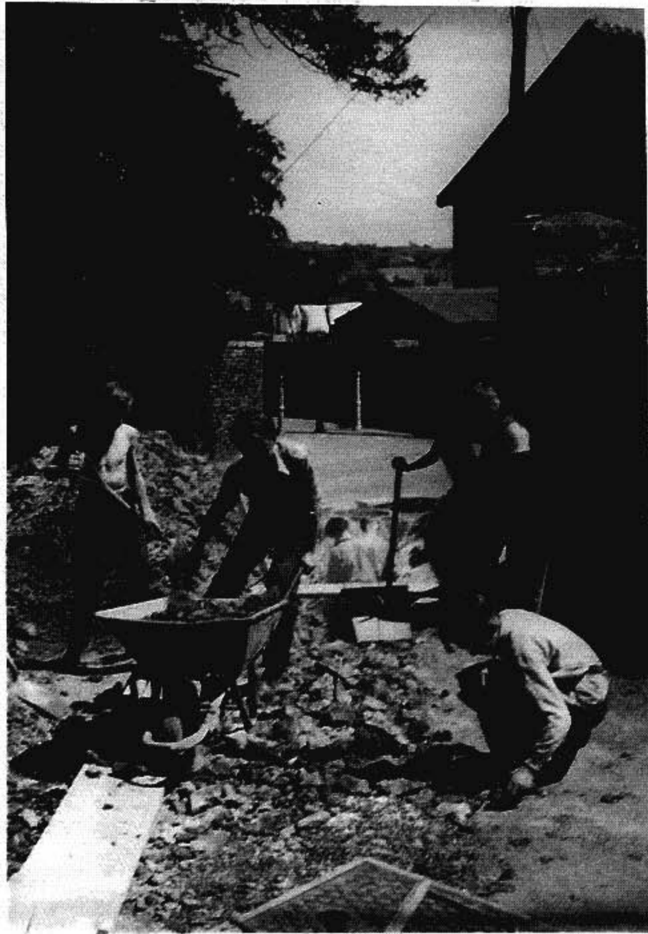
BACKFILLING UNDER WAY.
