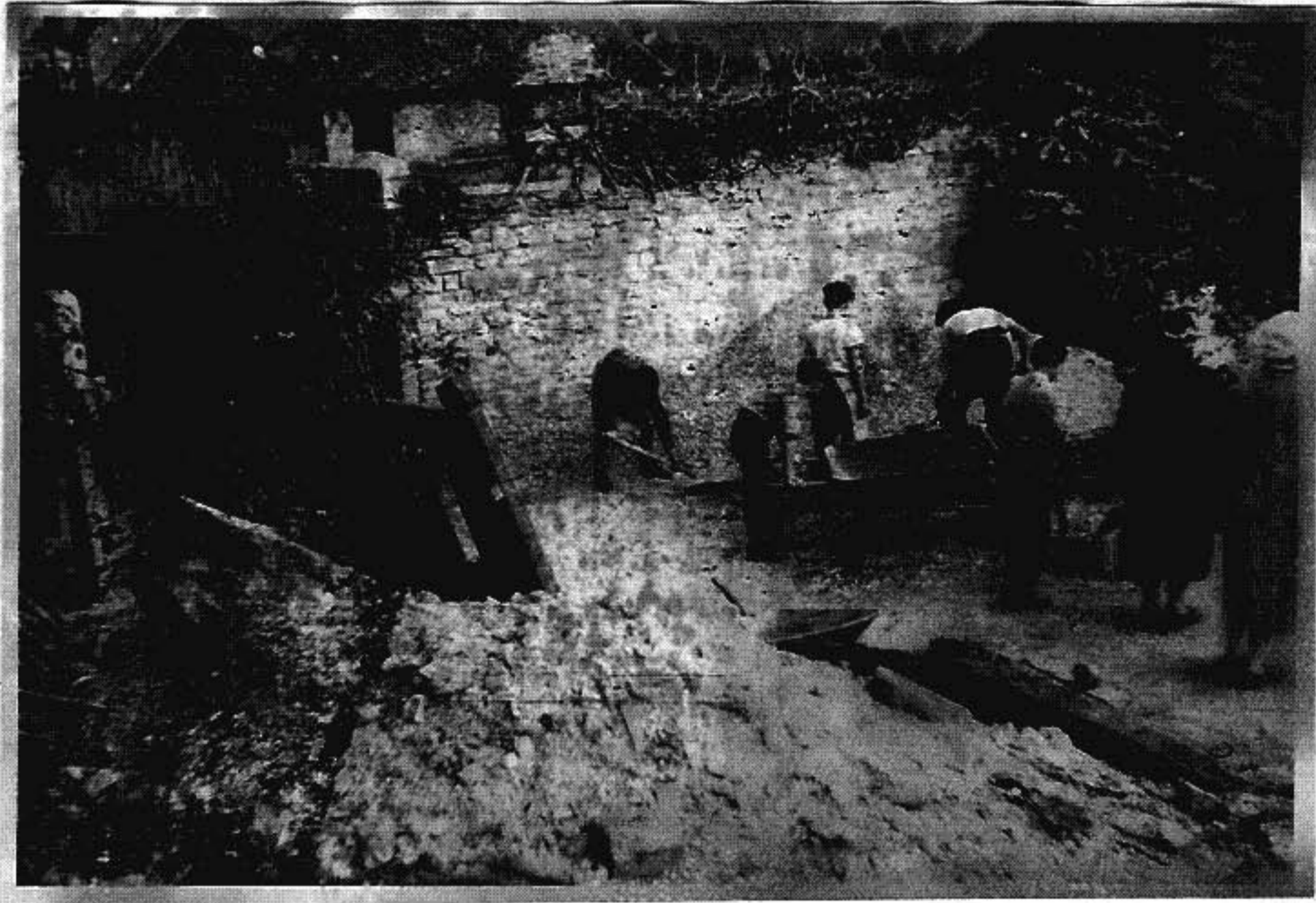
MECHANICAL DIGGING COMPLETED.
